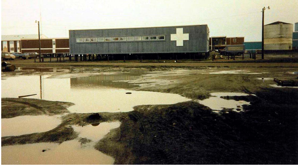
This hospital in Barrow, Alaska has been on the IHS facility list since 1991 and is in desperate need of replacement.
