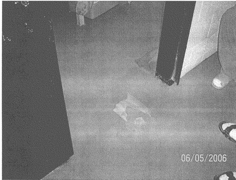
Reflecting lights in the sewage spill over
