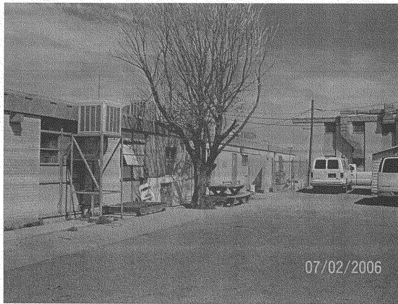
An overview of the exterior of a detention facility. Note the object in yellow, beyond the picnic bench, but in front of the green generator.
