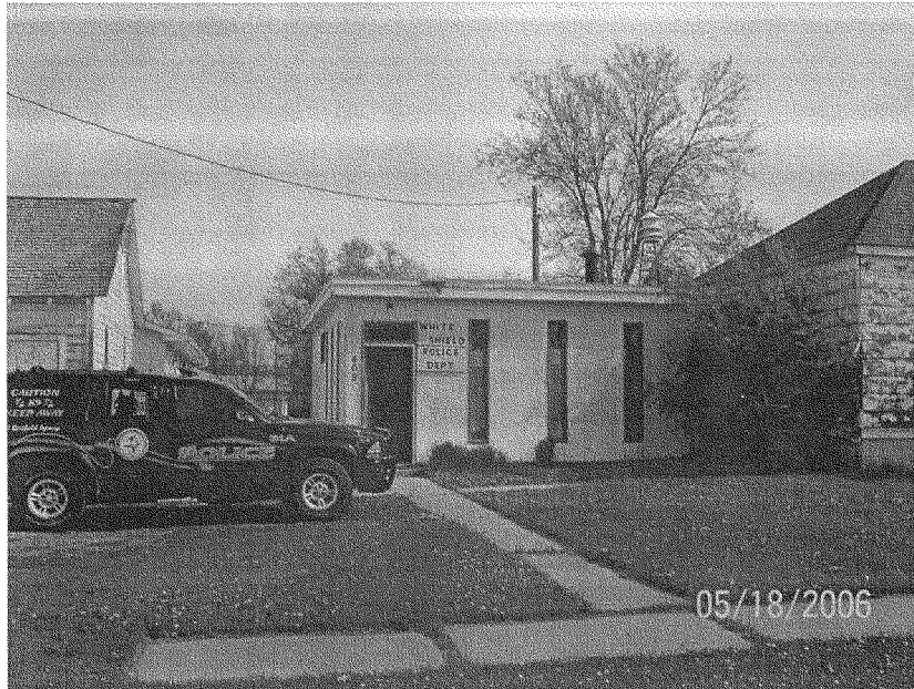
Building on left is used for evidence storage, the center building attachment is an operational Law Enforcement Substation with three cells, and the building to the right is the abandoned building that was used by the Bureau of Land Management
