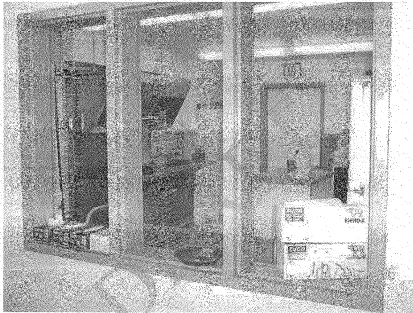
Free inmate access to the kitchen through the window with no window panes. Picture is taken from the common corridor used by inmates.
