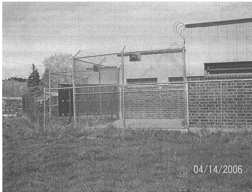
Because of the close vicinity, recreation yards may not be used for emergency evacuation as was stated at this facility
