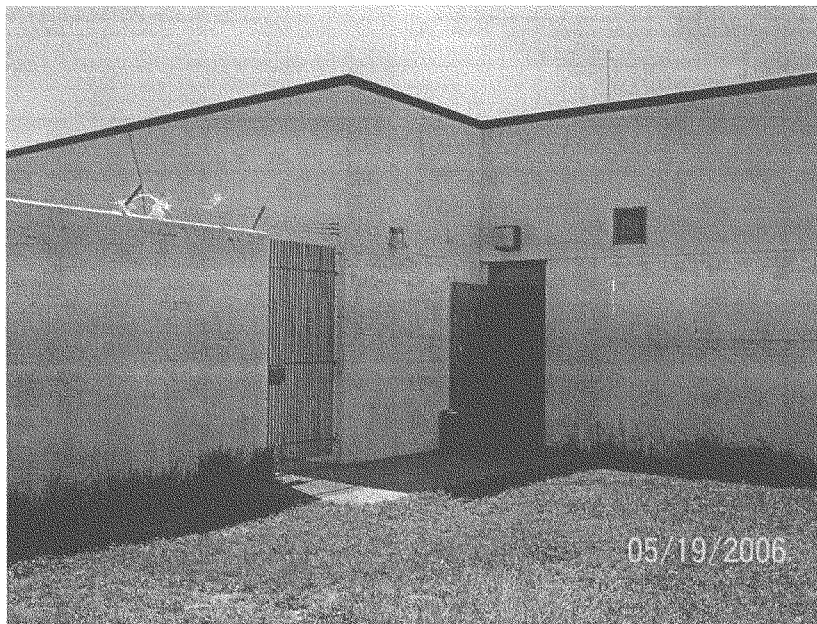
Gate in the recreation yard provides easy climb-out over the crossbars
