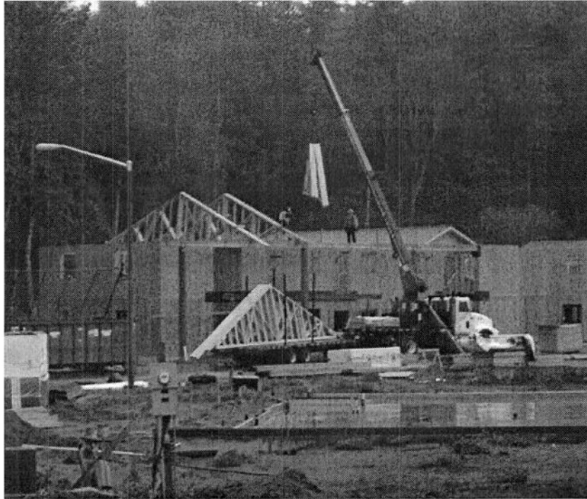
Kwina Village – Building foundations – Lummi Nation (Washington State)
