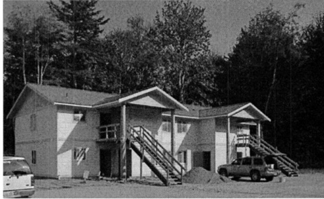
Kwina Village - One of the 9 apartment buildings nears completion.
