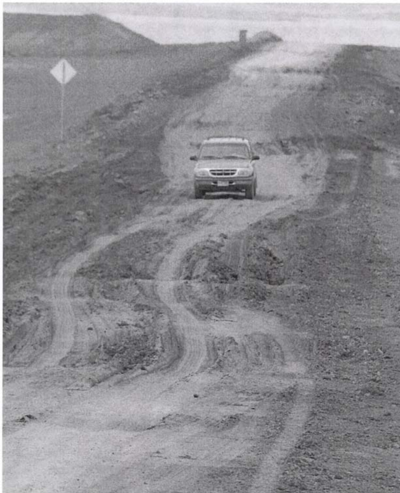
Photo of Oil and Gas Impacts on Fort Berthold Reservation Roads
