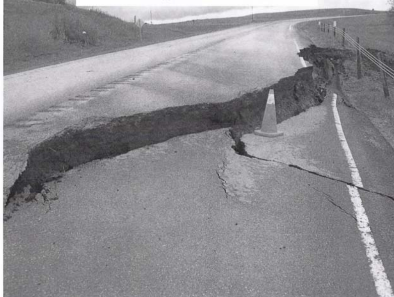
Photo of Oil and Gas Impacts on Fort Berthold Reservation Roads
